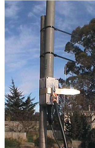
Fig. 21 Preamplifier slid up so that antenna pipe rests on the preamplifier
